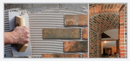
Interior or exterior mortar application on masonry or concrete.
