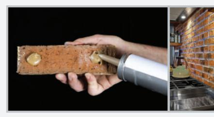
Adhesive interior installation on wood/steel stud framing.
